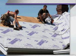
TITANIUM® PSU-30 ICE DAMMING PROTECTION
